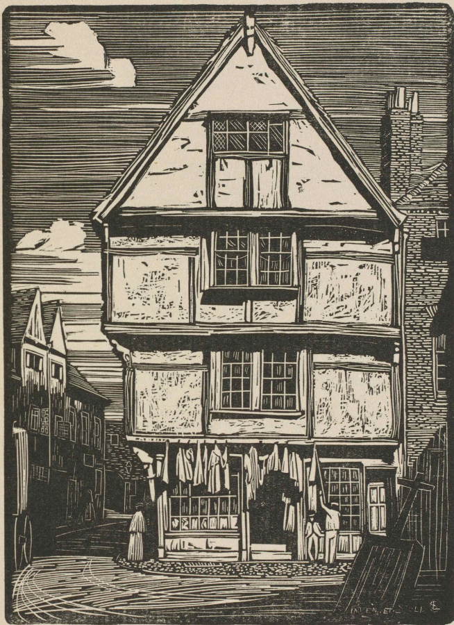
THE GABLED HOUSE.
